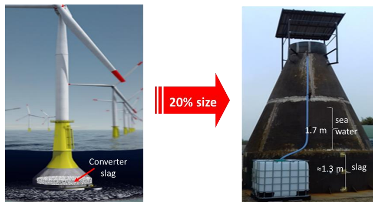
Figure 4: GBS selected design and steel prototype presentation
